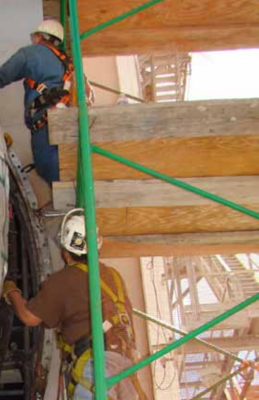
Various fabric expansion joints were installed at a waste incineration plant in Sweden, including a sealing joint between the furnace and the boiler.
